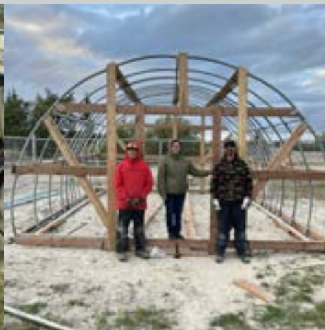
Building a greenhouse in Lac Brochet
